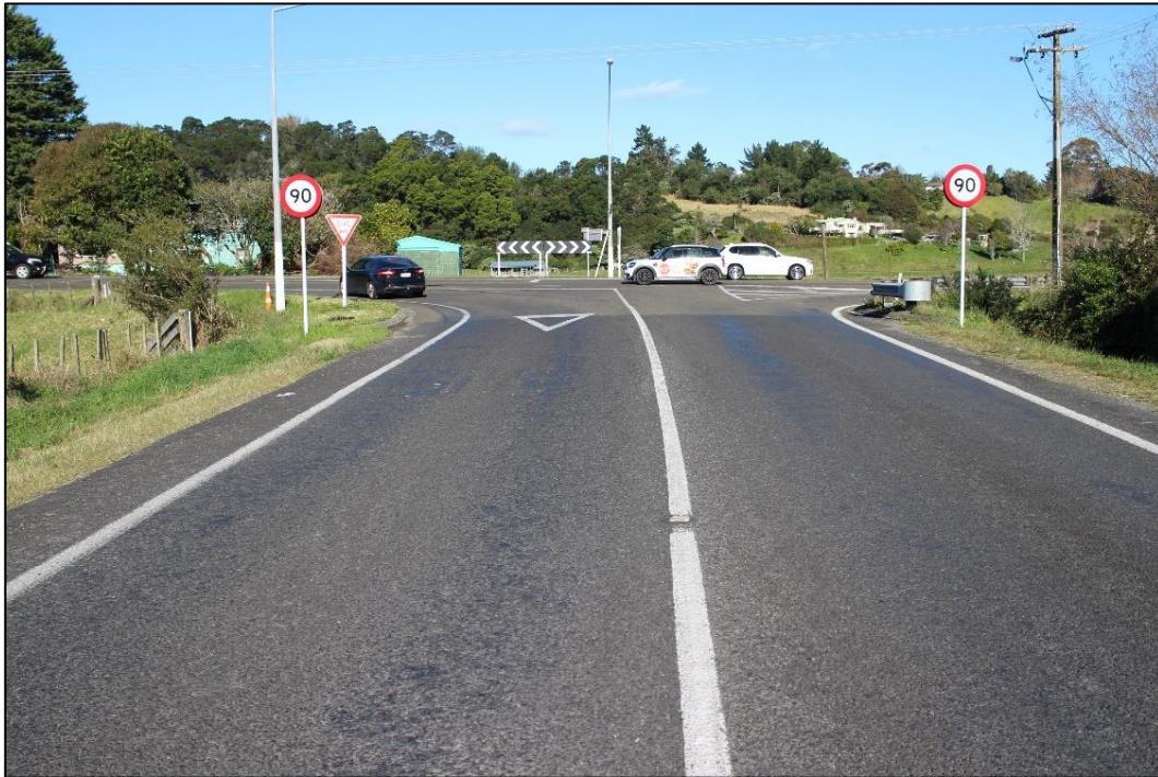
Photograph 4: Te Puna Station Road Approach to SH2
