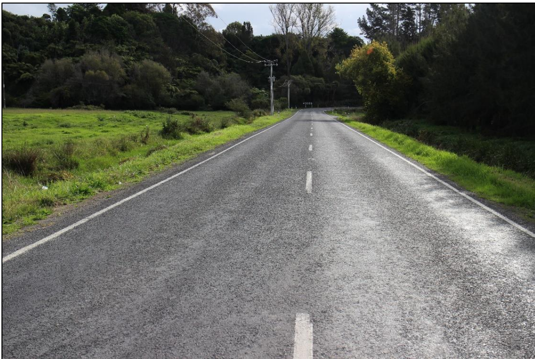
Photograph 3: Te Puna Station Road Looking West
