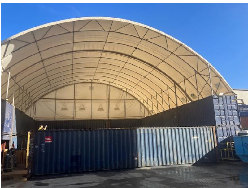
Figure 16 – Example Refurbishment Enclosure
