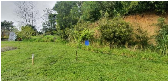
Photo 19 slope behind residential dwelling
