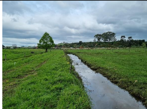
Photo 10 open stormwater drain looking east
