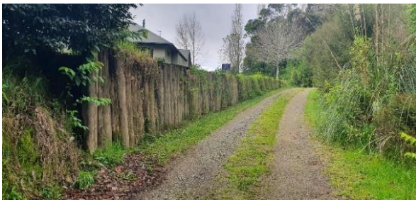
Photo 17 retaining wall on driveway
