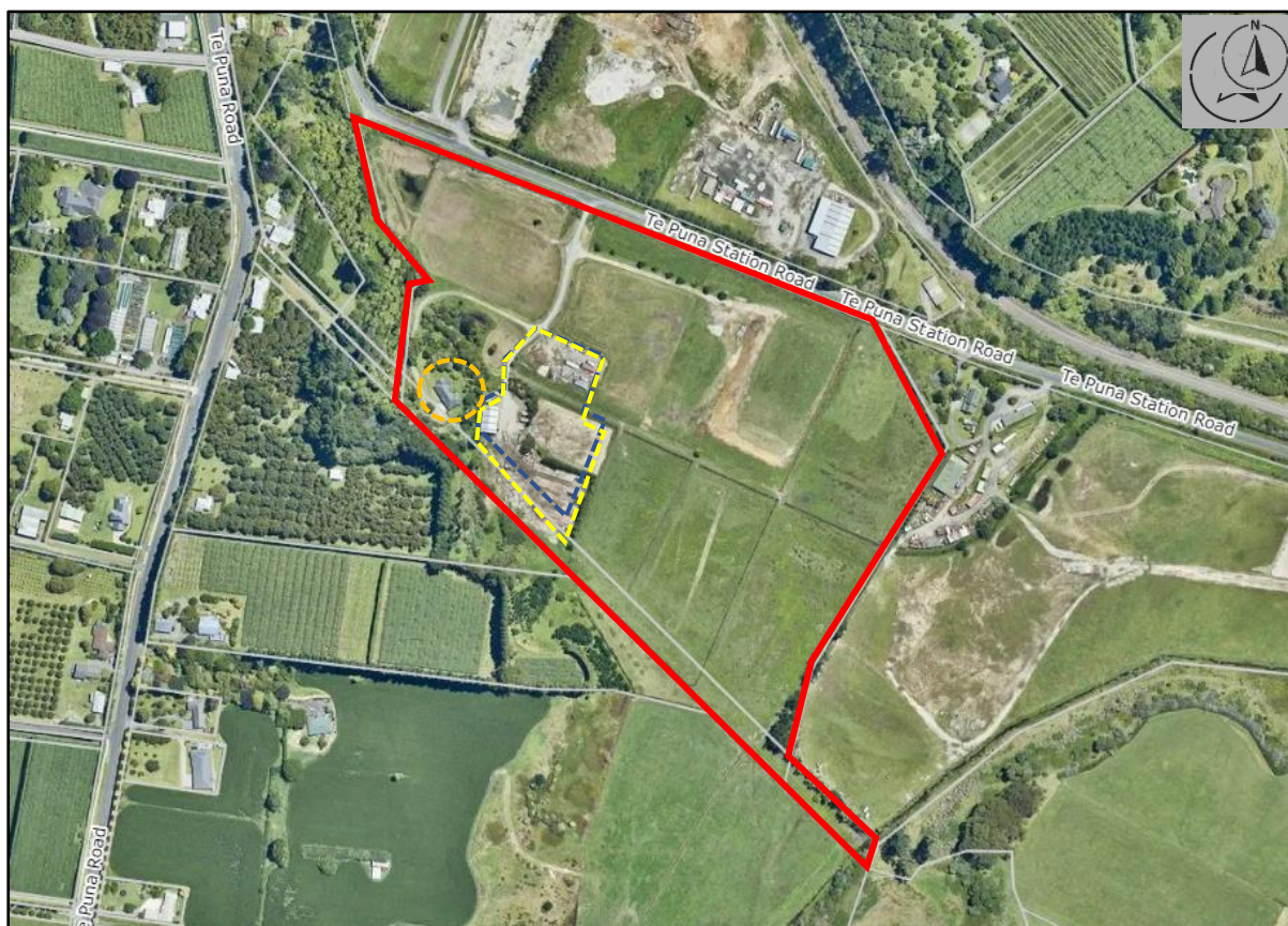
Figure 1: Subject site and existing features. The application site is bounded red. The existing dwelling is circled dashed orange and shed and associated yard spaces bounded in dashed yellow. Access is via a driveway in from the southern side of Te Puna Station Road, with secondary access routes across the site stemming from this driveway.
